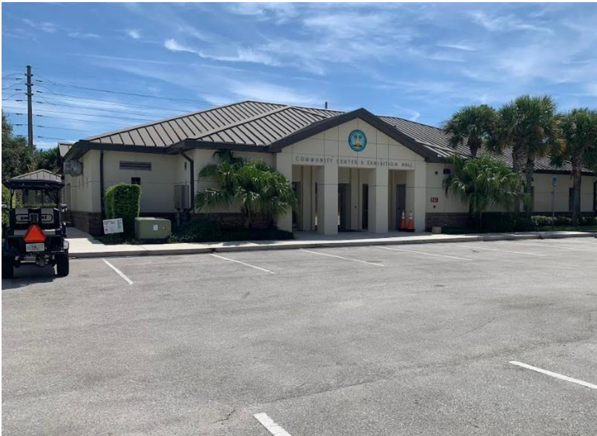
JACKSONVILLE BEACH COMMUNITY CENTER
